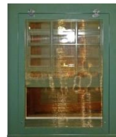
Metal Screen Mesh in Wood Frame with Exposed Metal Hangers
