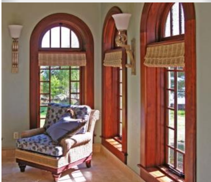
A hinged inswing screen is shown above in combination with a traditional pushout casement. Parrett also offers both automatic and manual rollscreen systems for pushout casements.
