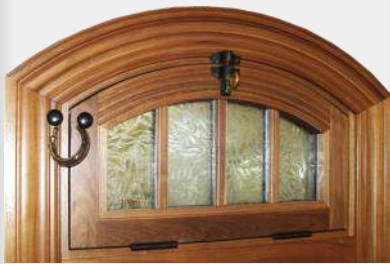
Traditional hopper with singlepoint latch/chain hardware shown above.
